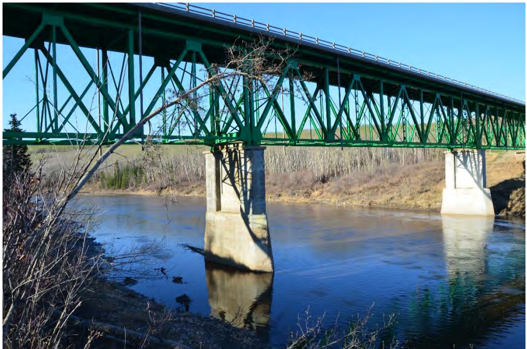
Bridge on Highway 49 over the Little Smoky River
